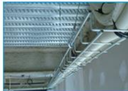
Refrigerant pipes
