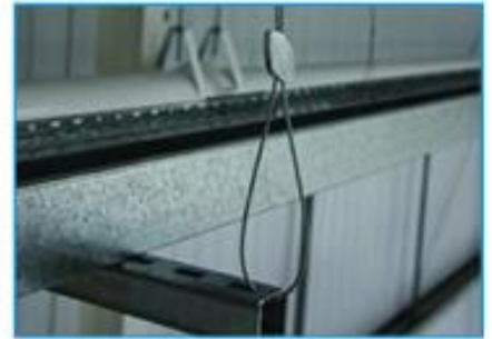
Perforated cable tray on channel
