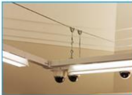
Lighting and Camera on Catenary
