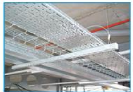
Multiple cable trays on single channel
