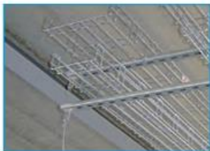
Multi-tiered cable basket on Trapeze
